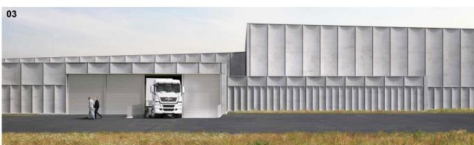
Danish Agro needed more storage space at Aarhus Harbour. The existing fertilizer storage hall was expanded by 2,500 m<sup>2</sup>. DS Flexhal also built a new hall of 8,000 m<sup>2</sup> divided into four sections and constructed with steel trusses. Precast concrete wall elements were supplied by DS Elcobyg and steel by DS Stålkonstruktion from DS Gruppen.
